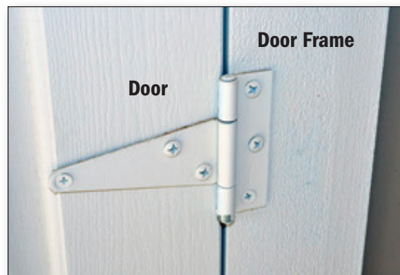
Shed hinges attached by simple screws to a shed exterior are vulnerable to burglars.
